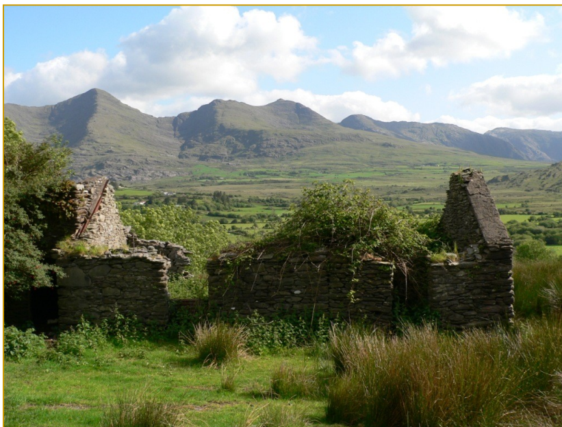
Abandoned farm building in Keas, Glencar
